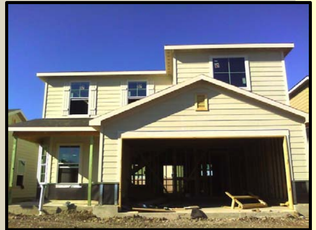
A picture of Norma Sanchez's (AT/A) House in Construction in May 2010.
